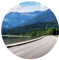
Roads, Bridges and Embankments
